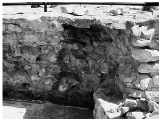
**Fig. 5.** Stone wall which cannot be subjected to hydrophobization (cracks, mortar holes, salinity)
